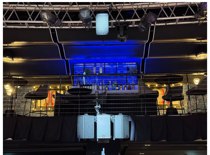
Rear Airsound Spatial array, featuring 4 Martin Audio CDD-8 Live units in a dipolar steering arrangement.
